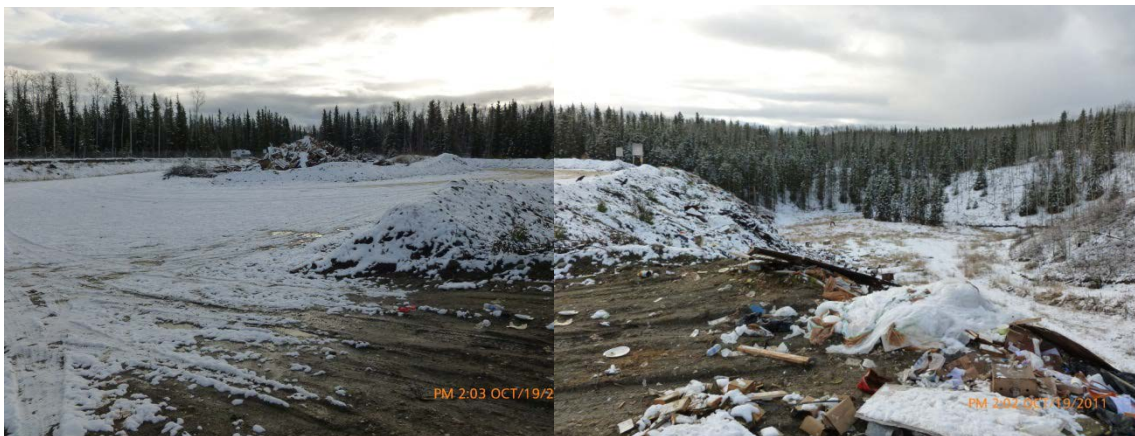
Photograph 6: Mayo Facility Waste Material; looking west to south.
