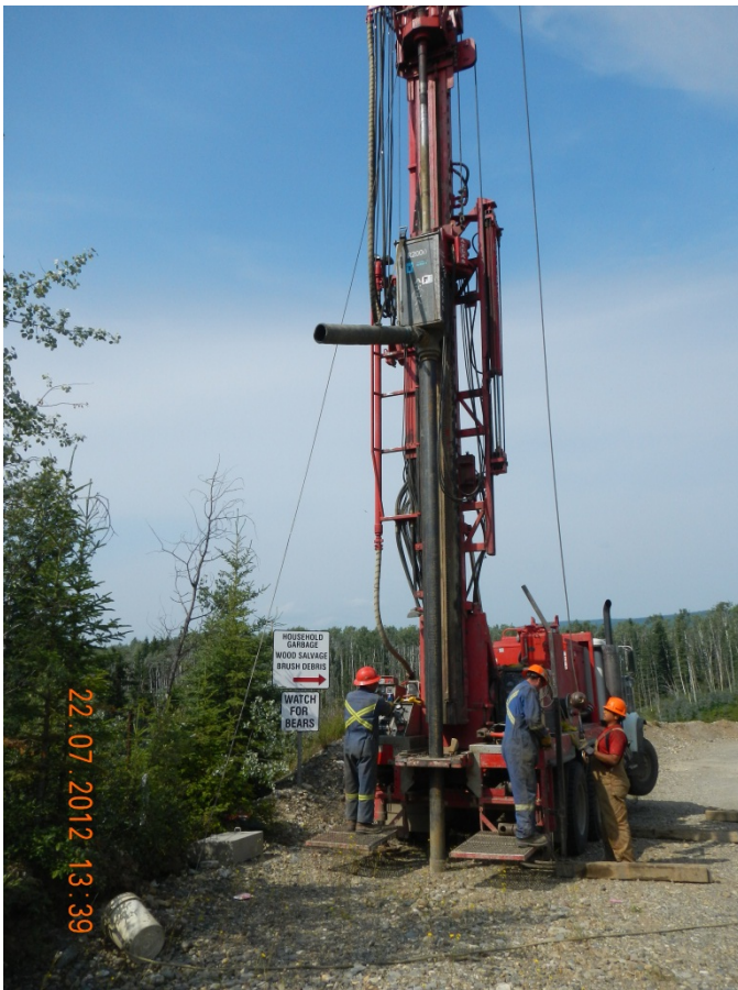
Photograph 5: Mayo Facility Drilling Well MA-MW12-01; looking north.
