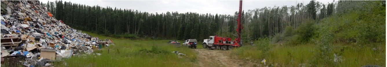
Photograph 3: Mayo Facility Drilling Well MA-MW12-04; looking southwest.
