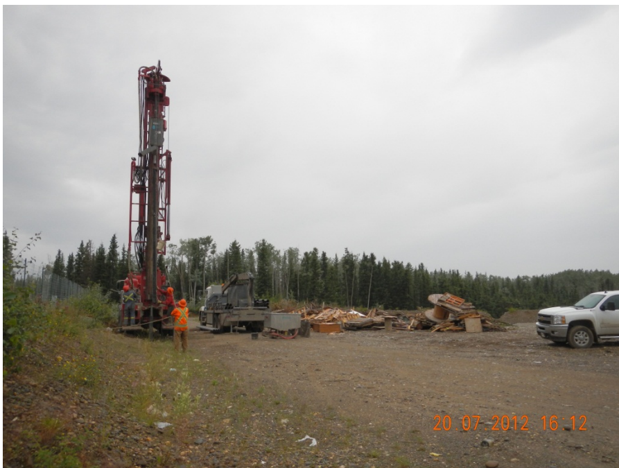
Photograph 2: Mayo Facility Drilling Well MA-MW12-02; looking north.
