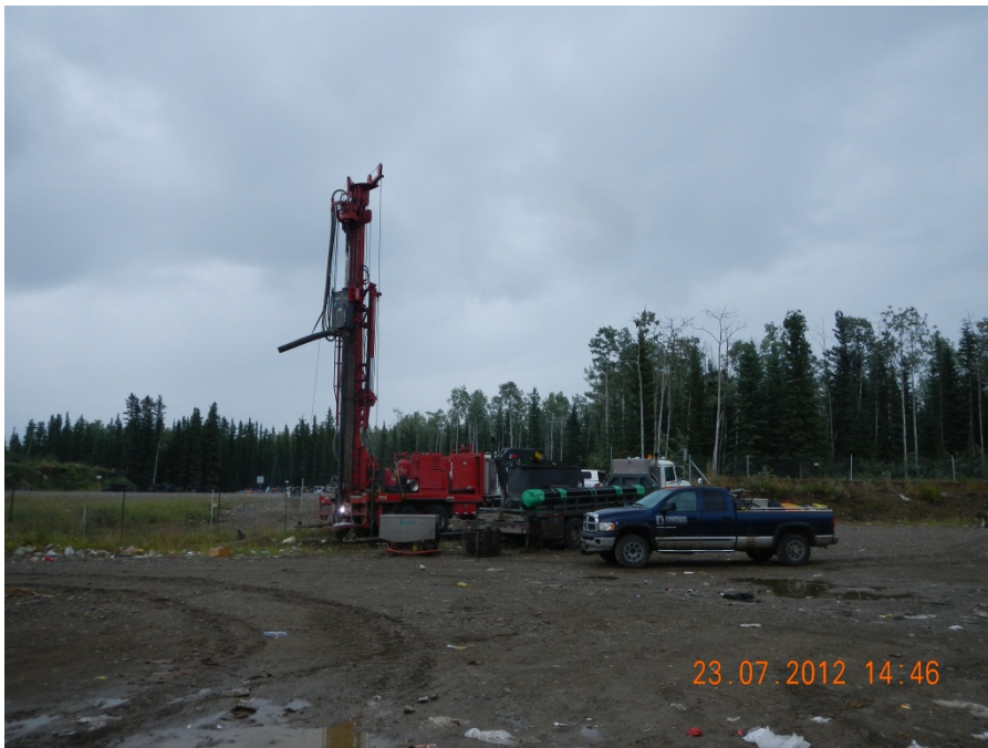
Photograph 1: Mayo Facility Drilling Well MA-MW12-03; looking northwest.
